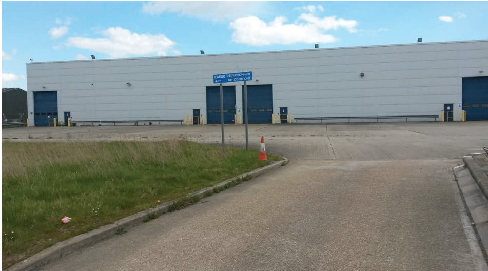
Existing Cargo Facility
