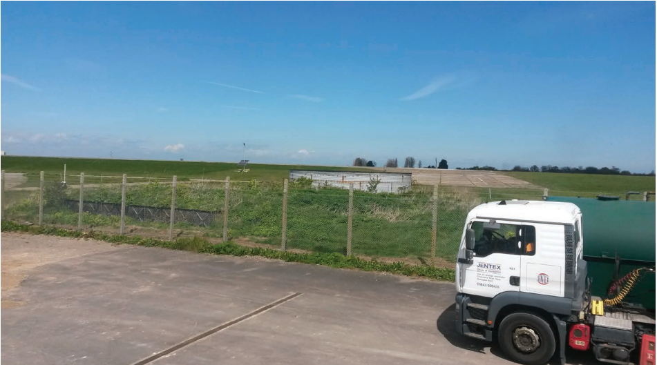
Jentex Oil Storage Depot
